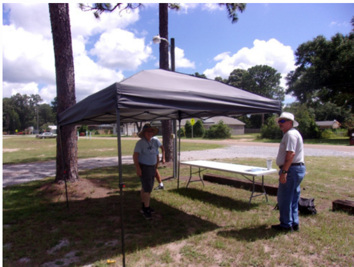
The installing of the protective canopy.
